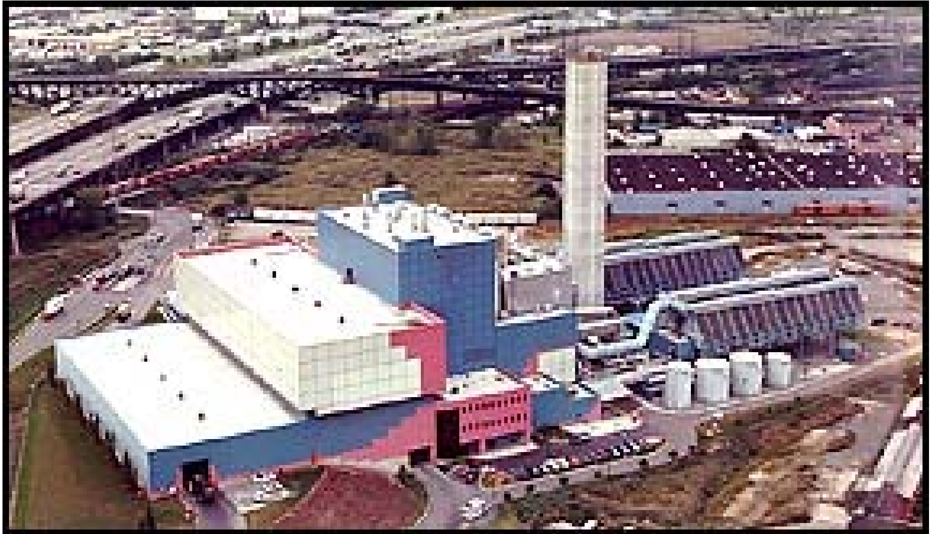
Essex resource recovery facility
